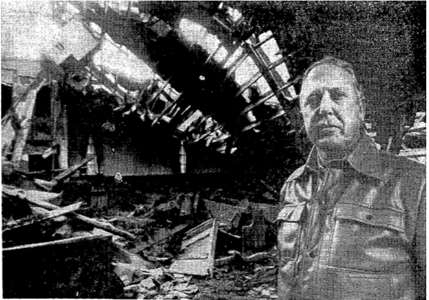
Rev. Guy Milam in church area damaged by fire.
